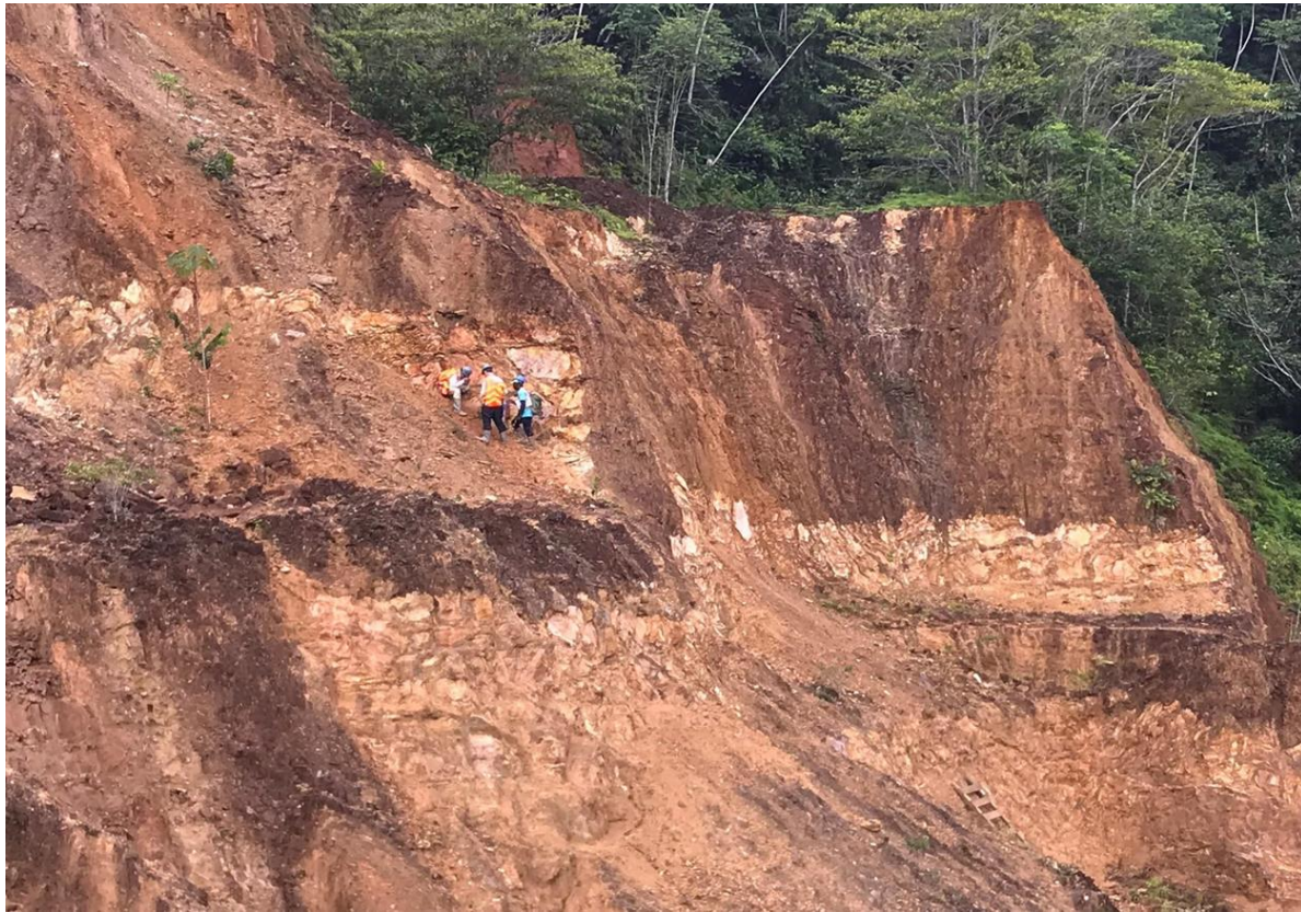
Figure 4. Photo of SJ prospect pit wall being cleaned for channel sampling.
